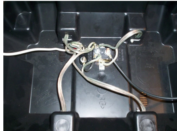
Inside view with circuit breaker in upper middle
